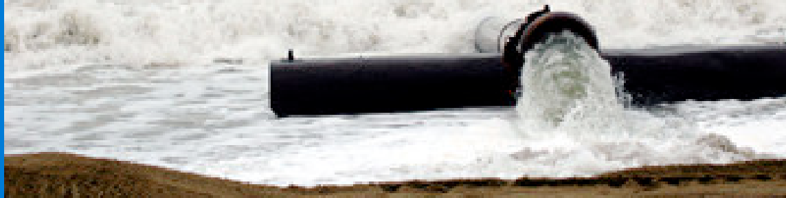
PIPELINE PUMPING WATER AND SAND
