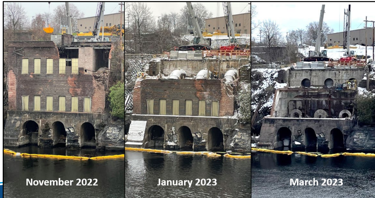
Powerhouse Deconstruction Progress
